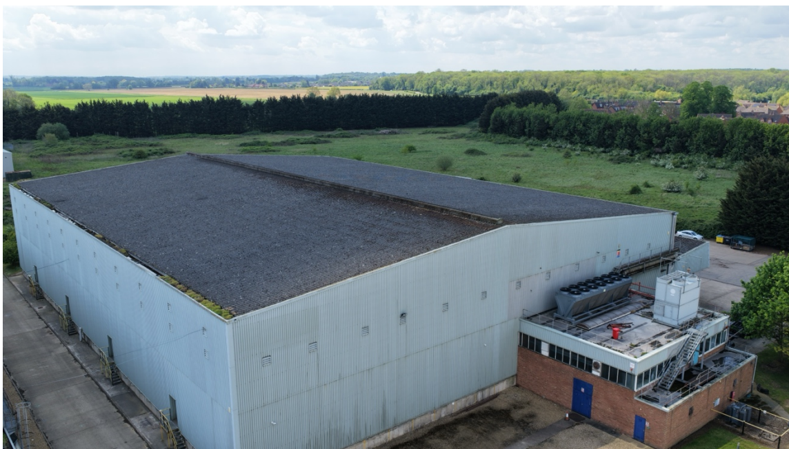
Figure 1. Aerial overview of the JS Davidson Bourne site roof areas.
