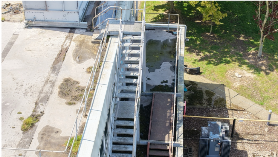
Figure 12. Water ponding
