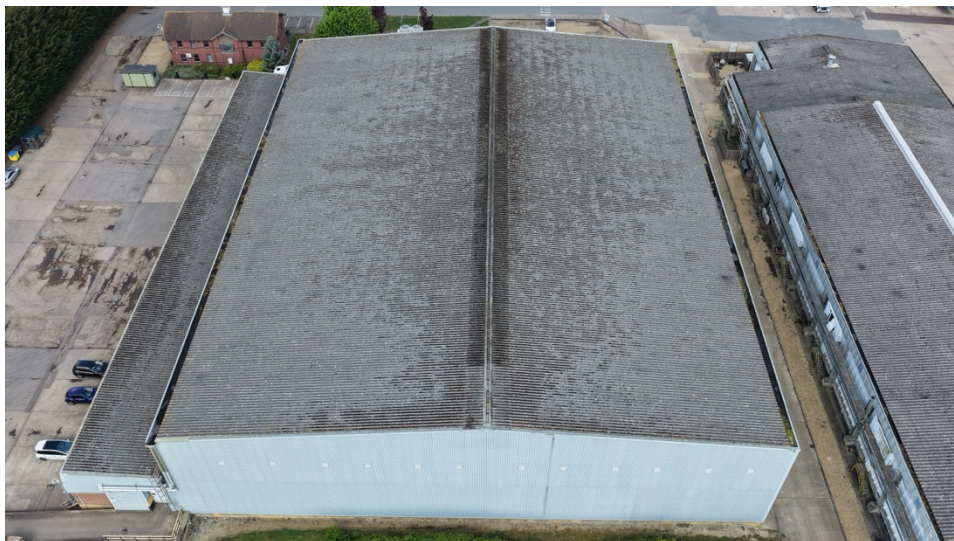
Figure 2. Oblique aerial view of the main warehouse roof.
