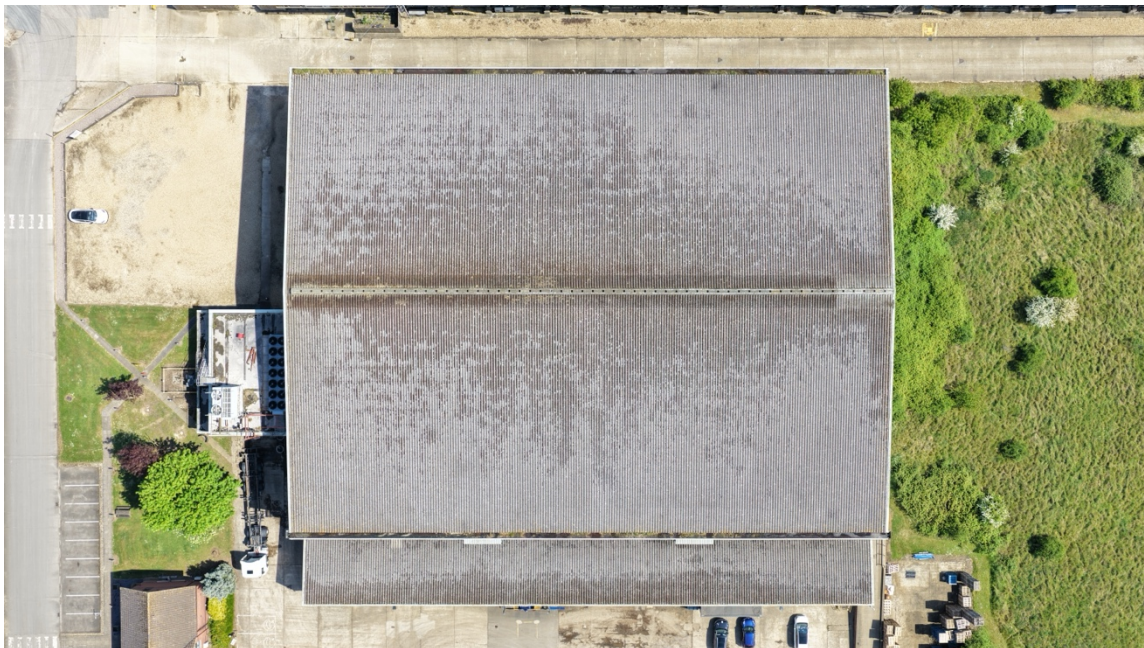
Figure 3. Aerial view of the JS Davidson facility illustrating the extent of the roof areas included in the inspection.
