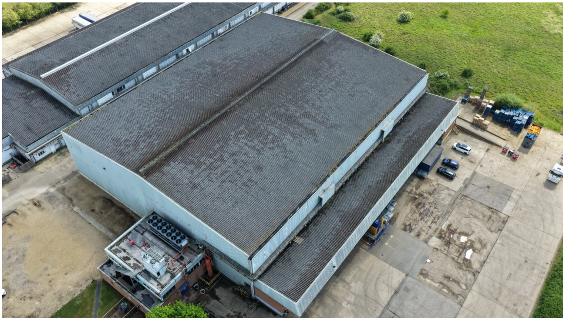
Figure 4. Oblique aerial view of the roof structure at the JS Davidson facility.
