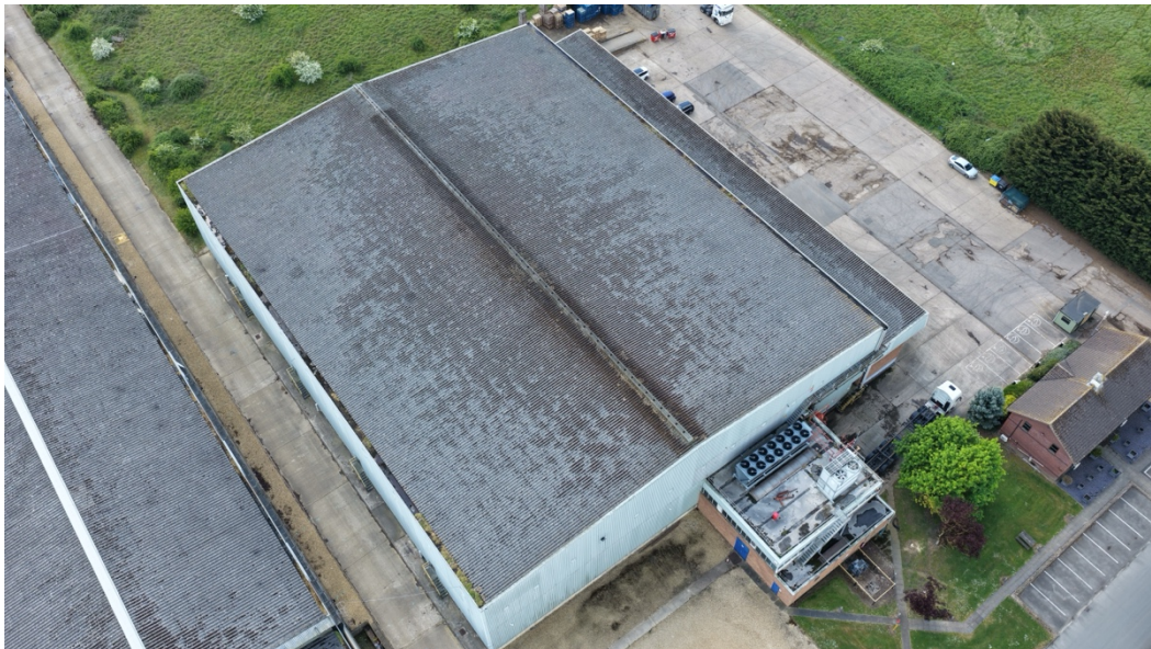
Figure 7. General Aerial Overview showing whole site.
