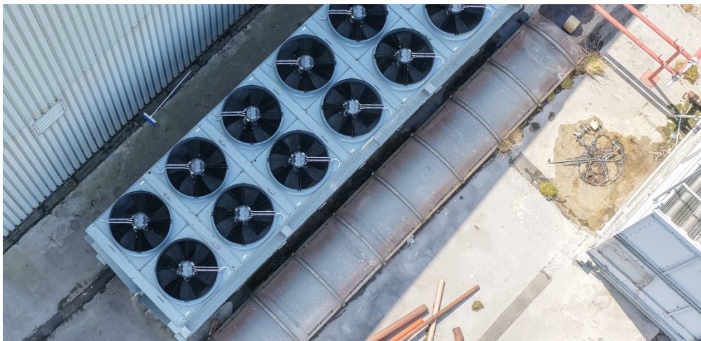
Figure 21. Weathered barrel rooflights with staining and moss/debris accumulation around adjacent junctions.
